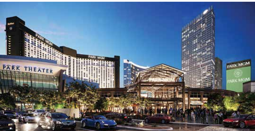
The construction, renovation and rebranding of the 2,700-room Park MGM is in its final phase, with some elements — including the boutique hotel NoMad — set to wrap up later this year.
