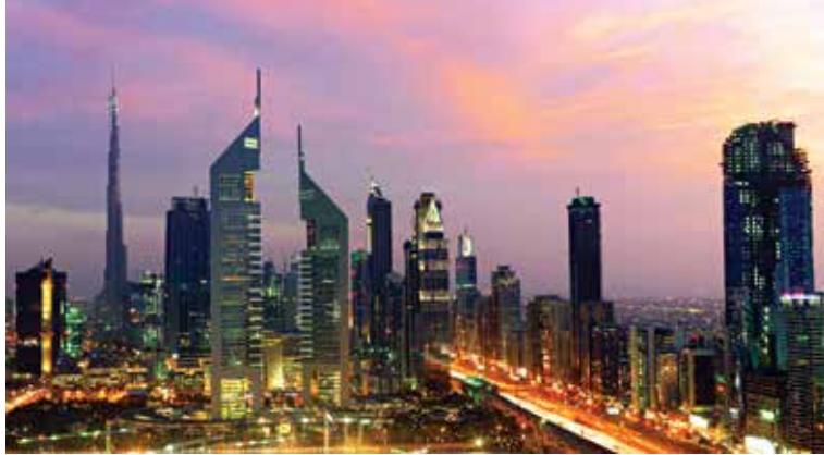
The triangular Emirates Towers in Dubai house a five-star hotel, office space and upscale shopping and dining.
